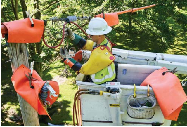
Penn Power lineworker Alex Greathouse installs an automated reclosing device on a single-phase power line in western Pennsylvania.
