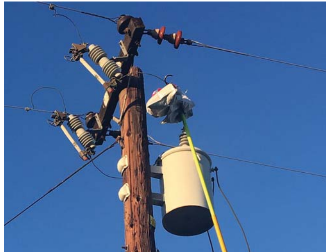
The balloons’ metallic coating is the conductor that leads to short circuits, outages and sometimes downed power lines.
