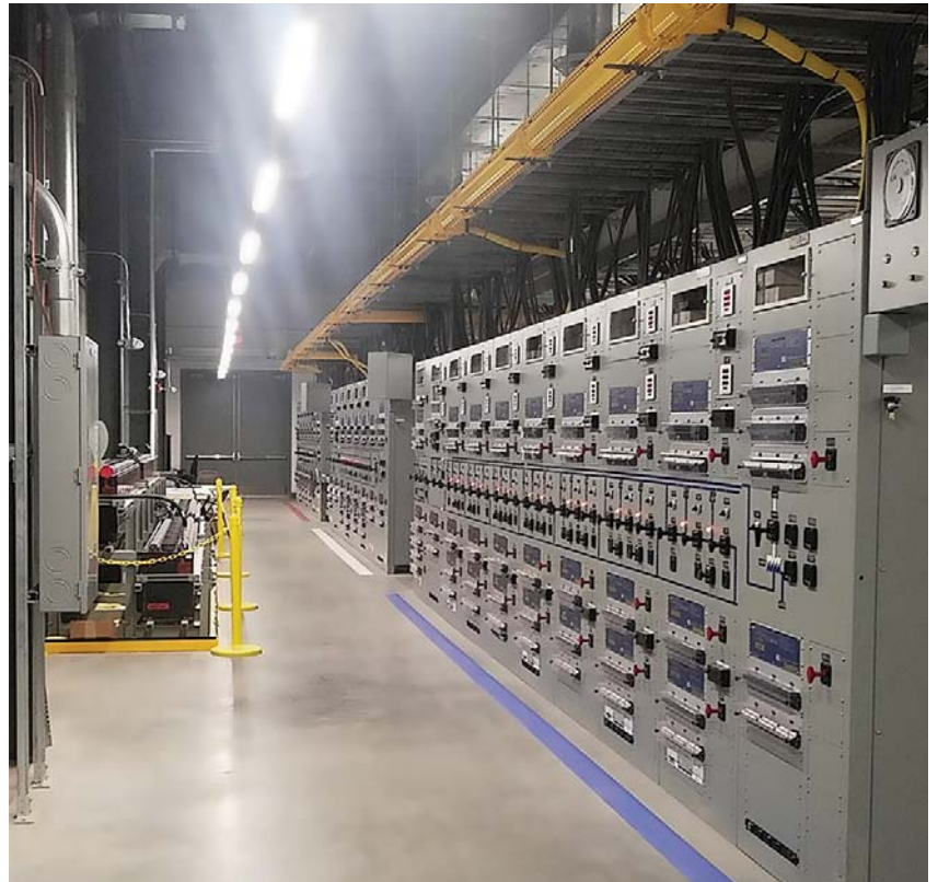
The building was designed to safely support the major equipment during normal operations and withstand system faults. The main switchboard control room is pictured here.
