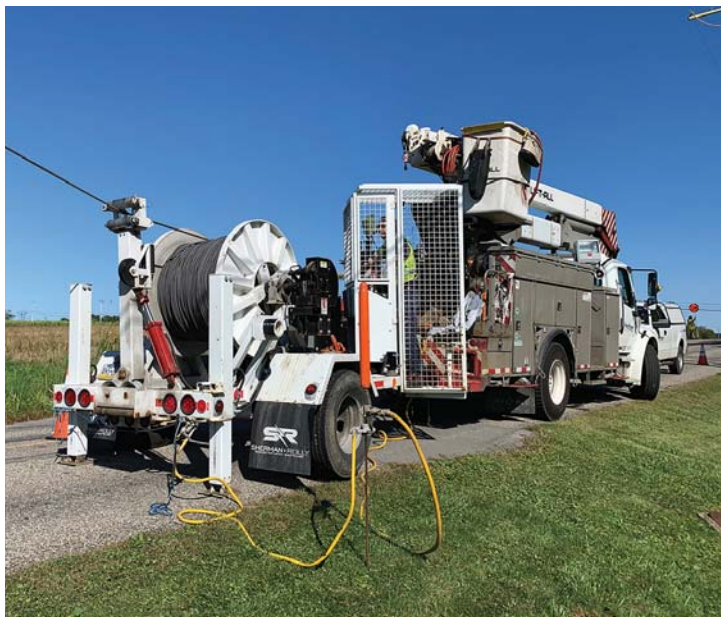
In the fall of 2019, Penn Power proactively replaced more than 184,000 ft of power lines with thicker, durable wire designed to withstand severe winter elements like ice and heavy, wet snow.
