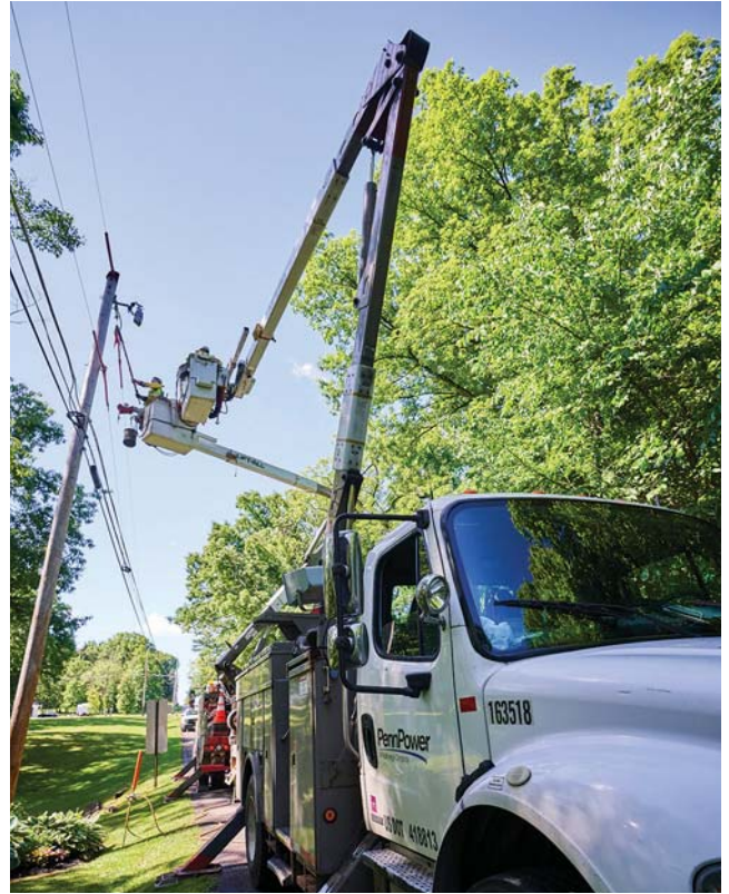
Penn Power customers will benefit from installation of new automated reclosing devices that can help restore power to customers within seconds in the event of a power outage and significantly reduce the length of an outage.
