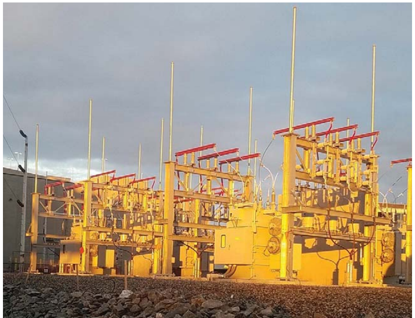
The outdoor yard housed three 115/11.5-kV power transformers and four 11.5/23-kV transformers.
