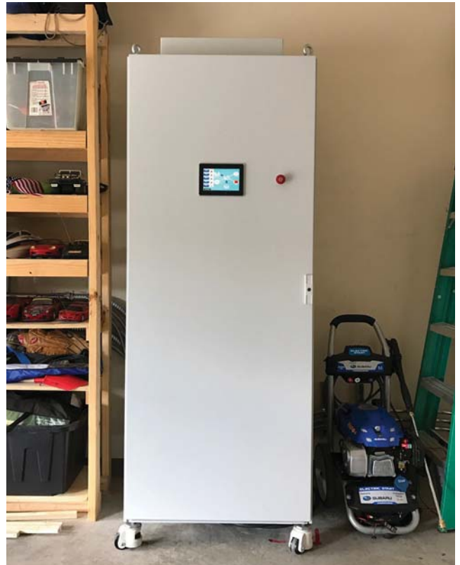
The Energy Switch is a complex system that includes energy storage and load control and monitoring.
