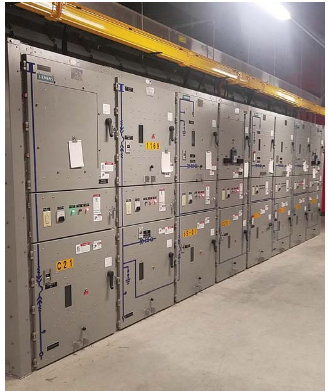
National Grid installed 63-kA rated arc-resistant switchgear manufactured by Siemens to replace the dated breakers and protection scheme in the old substation.
